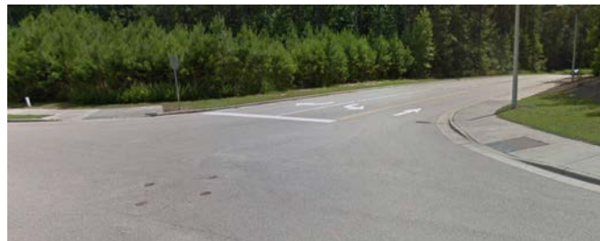
Lake Myra Elementary - Lack of crosswalk
