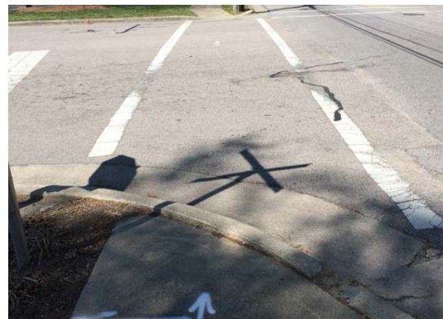
Wendell Blvd & Pine St - Lack of ramp access to crosswalk
