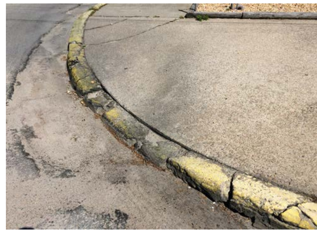
Cypress St & Third St - Lack of ramp access to sidewalk
