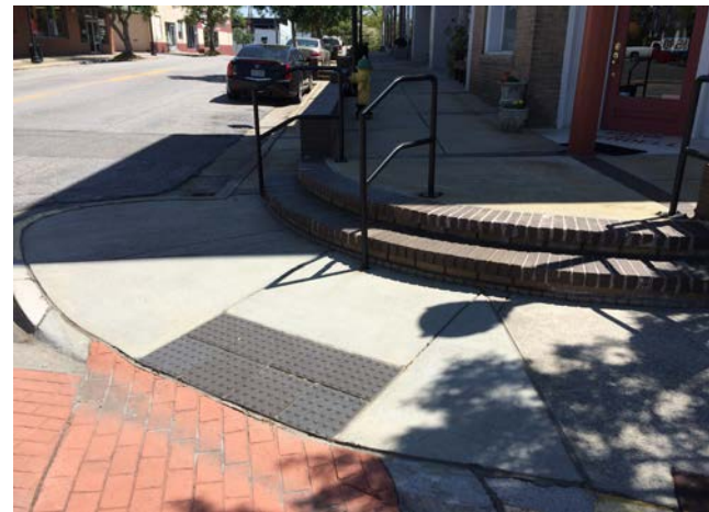
Main St & Third St - Ramp access present to stairs
